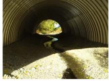
Photo on left shows current perched culverts on downstream side of West Beach Creek. These culverts were removed in October 2014 and replaced with one sixteen foot culvert, shown right, allowing fish to pass unobstructed. Good news: June 2015 monitoring activities documented a 3-4 inch salmonid approximately 100 feet upstream of the new culvert.
